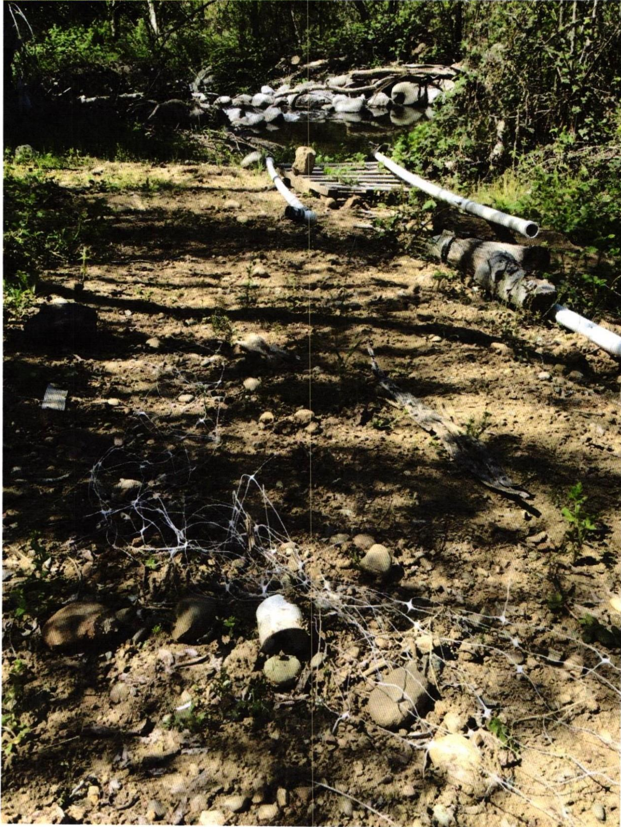
Figure 5: Access road to stream channel, eroding and discharging sediment to the stream. Diversion infrastructure and miscellaneous rubbish laced a/on the stream channel.
