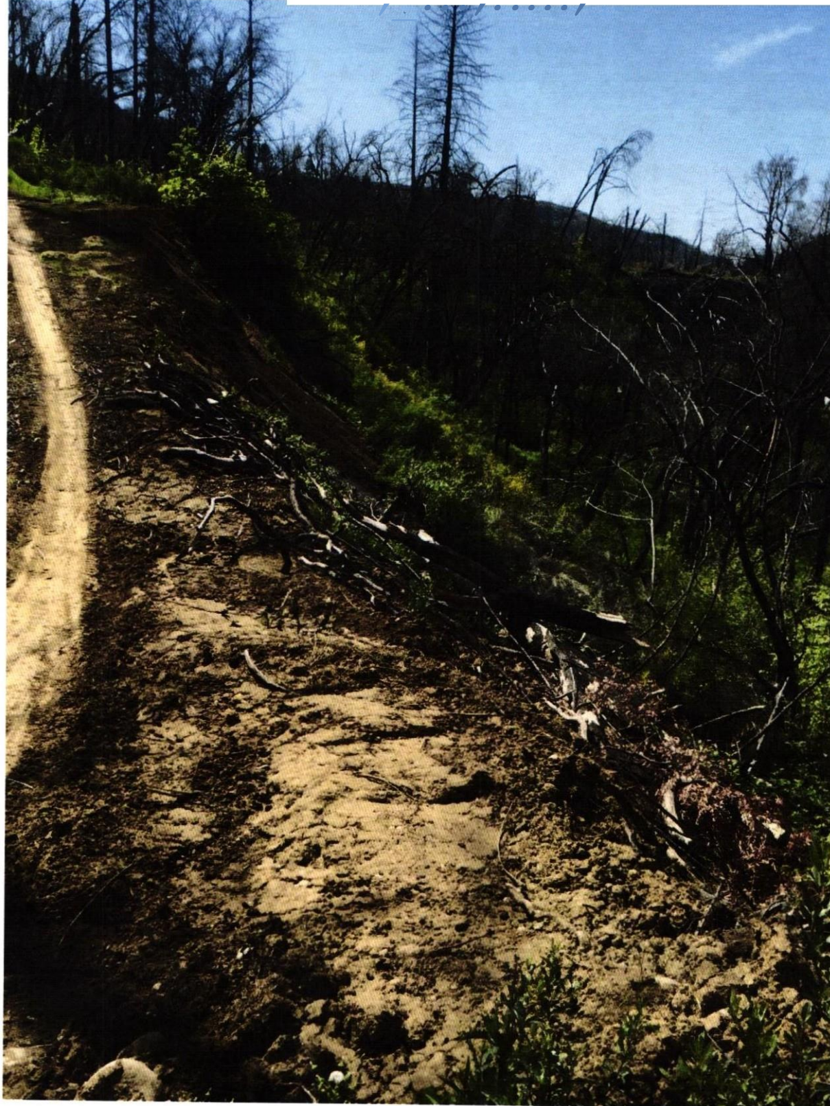
Figure 3: Sidecast sediment and woody debris discharged from road surface.
